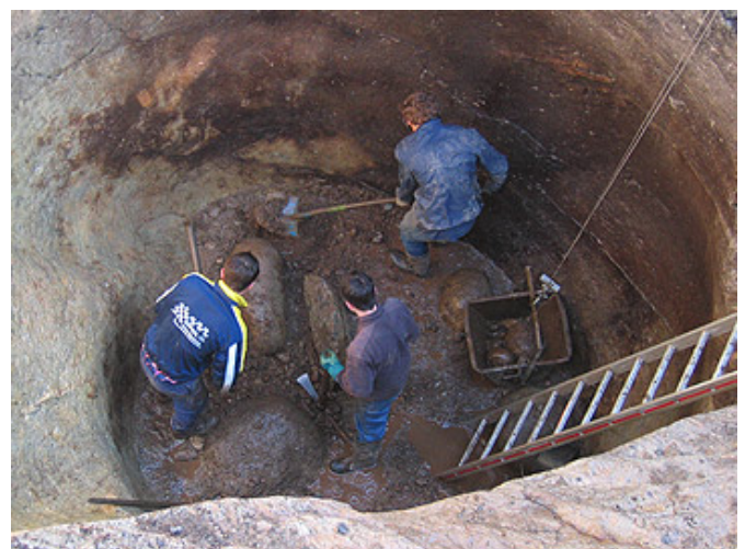
Emptying of a pothole
